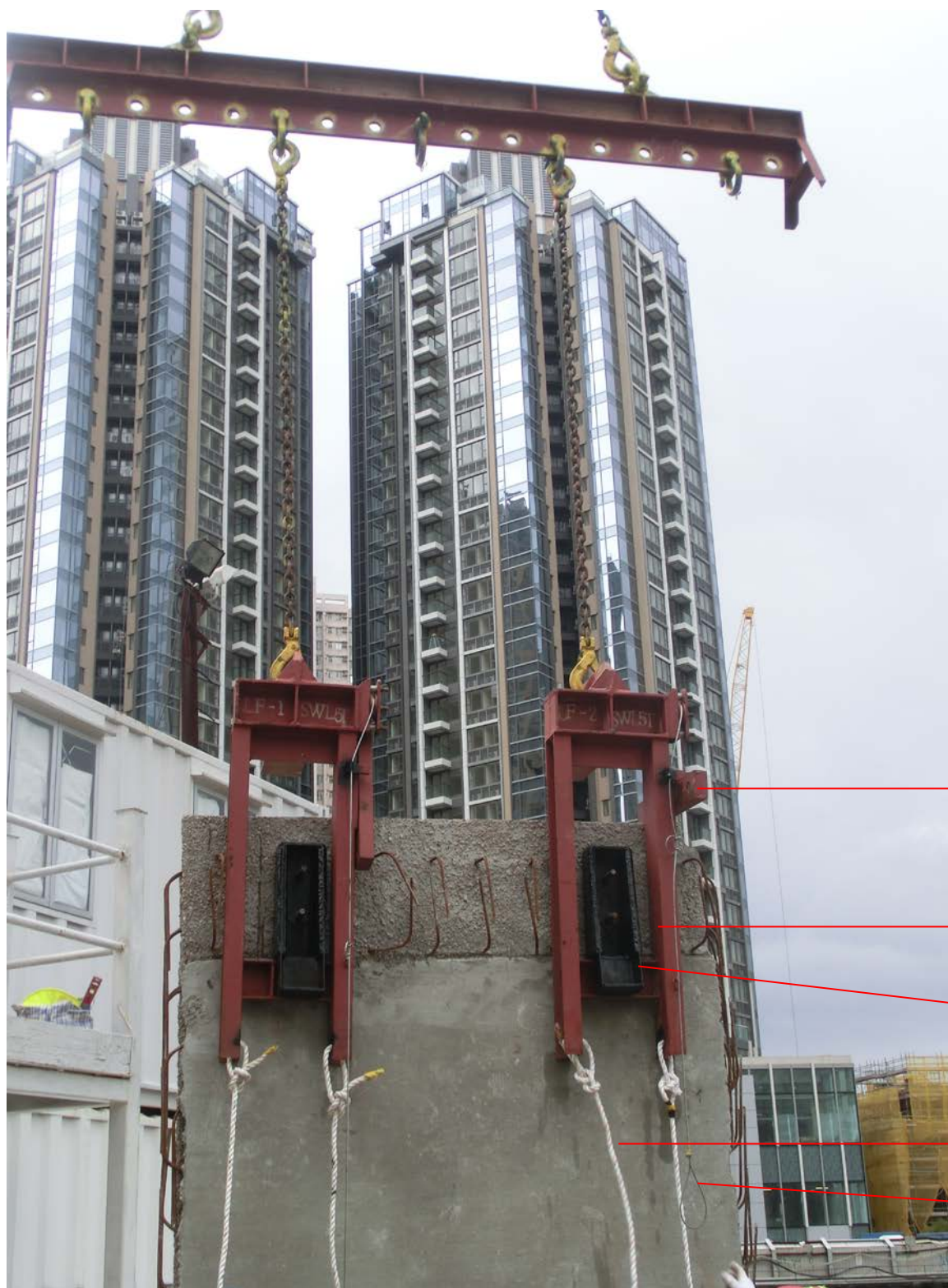
A New Way for Precast Facade Lifting (Lift-bolt Clamp)
